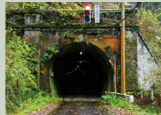
4 Iradani Tunnel (467m)
