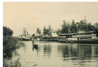
The Former Nagahama Port (1912)
