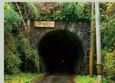
10 Sorojidani Tunnel (401m)
