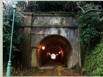
14 Kashimagari Tunnel (87m)
