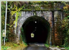
8 No. 1 Kannonji Tunnel (82m)
