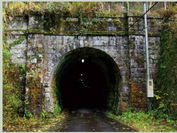
6 Magaridani Tunnel (260m)
