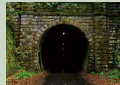
7 No. 2 Kannonji Tunnel (310m)
