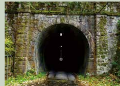
5 Ashitani Tunnel (223m)
