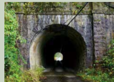
11 Funagaya Tunnel (64m)
